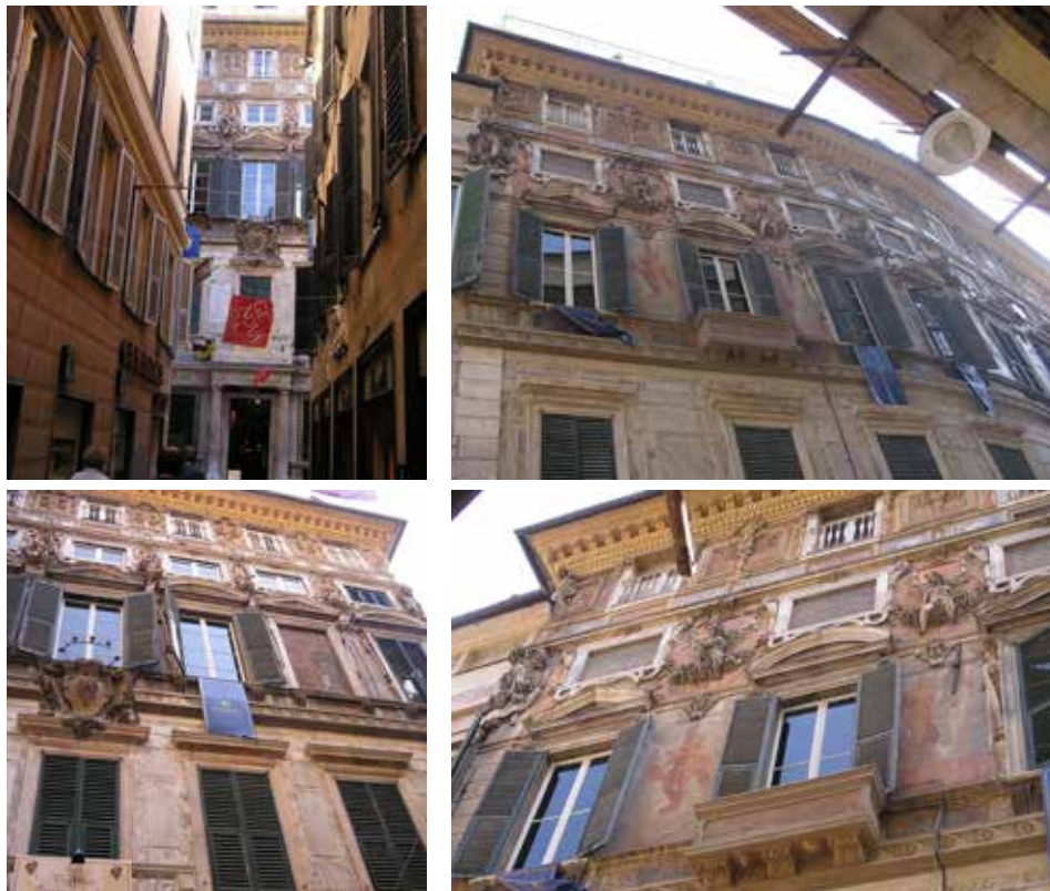
Fig. 20 Façade with plaster decorations and painted panels which still characterize the square. General and details view.
