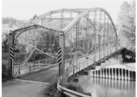
Fig. 8b 1858: construction of the Royal Albert bridge. Fig. 8c 1888: Ouaquaga Lenticular Truss Bridge built. It is composed of two identical lenticular trusses with an overall length of 105 m. [Historic American Engineering Record; Library of Congress HAER NY,4-OUAQ,1-3]. Pons Ligneus is similar also to Bardwell's Ferry Bridge, built in 1882, a lenticular truss bridge spanning the Deerfield River in Franklin County, Massachusetts.
