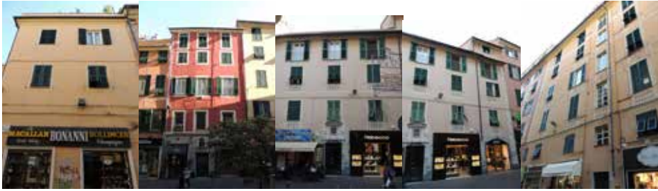
Fig. 5 via San Vincenzo. Prospects of apartment buildings; it should be noted, in particular, the unusual presence of the distribution system in the facade, easily recognizable by the “poor” treatment of the openings, without external fixtures.
