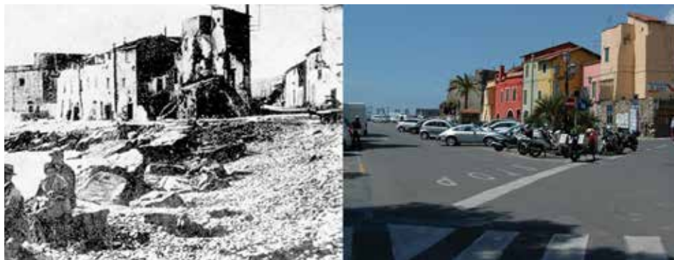
Fig. 4 The tower of Riva Ligure: a comparison of a photograph of the early twentieth century and a current photograph
