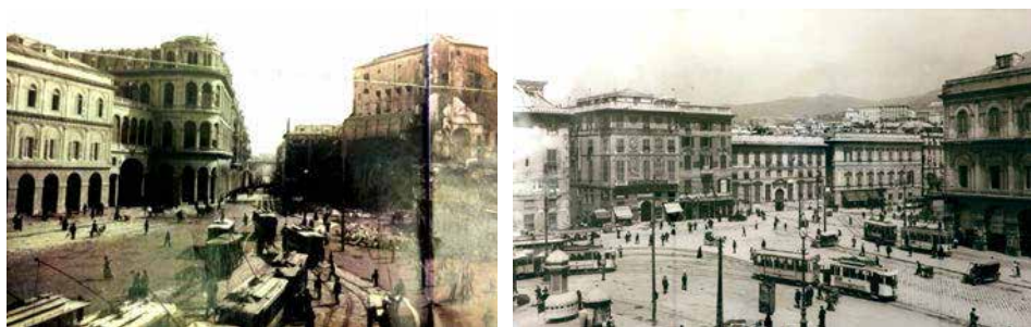
Fig. 28 Cartolina. Postcard. Demolition works of the Convent, De Ferrari Square and the new buildings of Via XX Settembre. Fig. 29 On the right some painted facades still preserved.
