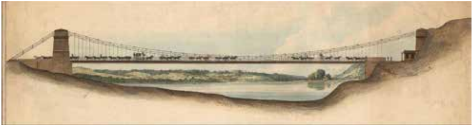
Fig. 4 The Union Bridge (1819-20) crossing the River Tweed between Horncliffe, Northumberland, England and Fishwick, Berwickshire, Scotland, built by Captain Samuel Brown. This wrought iron suspension bridge with iron chains has a single span of 137 m. [Drewry, 1832; p. 37-41].
