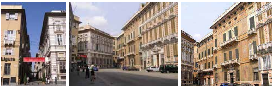
Fig. 34 The rich chromaticity of the square, and in particular the painted facade of the preserved Pallavicino Palace, strongly characterizes this urban space.
