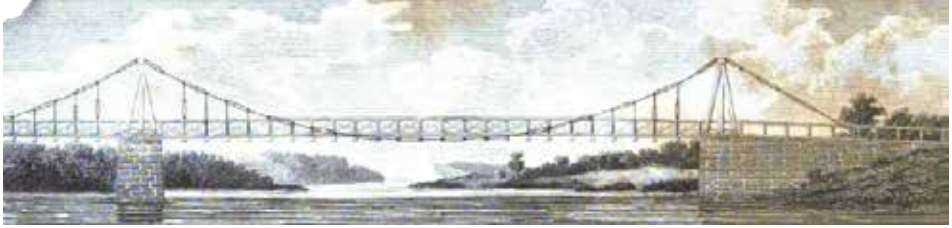
Fig. 3 “View of the Chain Bridge invented by James Finley” also known as Chain Bridge at Falls of Schuylkill, Philadelphia, Pennsylvania (1808) [The Port Folio vol. 3, no. 6 (Philadelphia: Bradford & Inskip, June 1810), p. 441-453 (original from Harvard University)]. The Jacob’s Creek Bridge was the first suspension bridge with iron chains (span length 21 meters, 3.81 meters wide deck).
