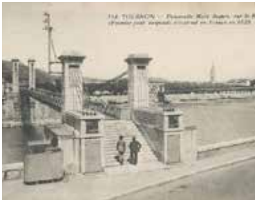
Fig. 6a This bridge, consisting of two spans of 85 m. each, linking Tournon-sur-Rhône to Tain-l'Hermitage, put into service on 25/8/1825, was actually the first large suspension bridge in continental Europe. The bridge, suspended by eight iron cables, has a total length of 170 m. [Cotte, 1986]. Fig. 6b Elevation and plan of the bridge on the Garigliano (1832), Luigi Giura design (1826); see: Di un nuovo ponte sospeso a catene di ferro sul Garigliano in Annali Civili del Regno delle Due Sicilie T. 1. Napoli: Dalla Tipografia del Real Ministero degli Affari Interni, 1833; p. 41-51 (span length: 80.40 m.s.; wide deck: 5.50 m.) .
