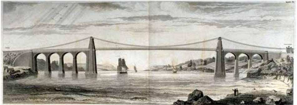
Fig. 5 Menai Suspension Bridge from Life of Thomas Telford, civil engineer. Ed. by John Rickman. London: Payne and Foss, 1838. The Menai Bridge was the first important modern suspension bridge with a span of 176 meters. The deck was suspended by sixteen iron chains, each composed of 935 iron bars, for a total of 2,000 tons of wrought iron, from two masonry towers at either end.
