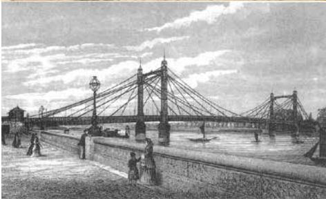
Fig. 11a Pons Ferreus, cable-stayed bridge with a tie rods anchored to masonry towers system. Fig. 11b 1873: Albert Bridge in the Illustrated London News. Fig. 11c 1891: Bluff Dale Suspension Bridge.
