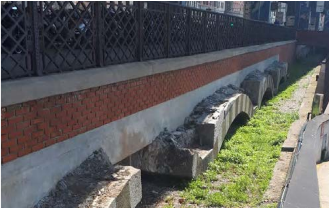
Fig. 7 Traces of ancient piers, difficult to be understood today
