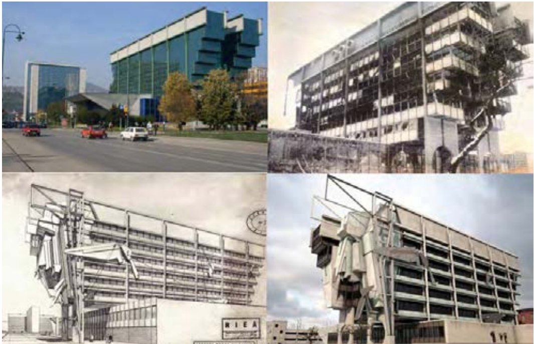
Fig.6 Electrical Management Building in Sarajevo: before the war (Ivan Straus 1978), the building destroyed by the war (1993), Lebbeus Woods project (1984), Computer rendering by Carlos Fueyo (2004)
